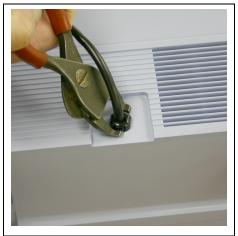
FIGURE 8-4: STRAIN RELIEF REMOVAL
